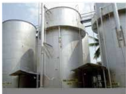
Figure 16. Anaerobic reactors for the treatment of rice mill effluent. Picture 1 shows plant under construction. Picture 2 show heat exchangers for cooling parboil mill effluent. Picture 3 shows gas driven backwash system in new generation anaerobic reactor.
