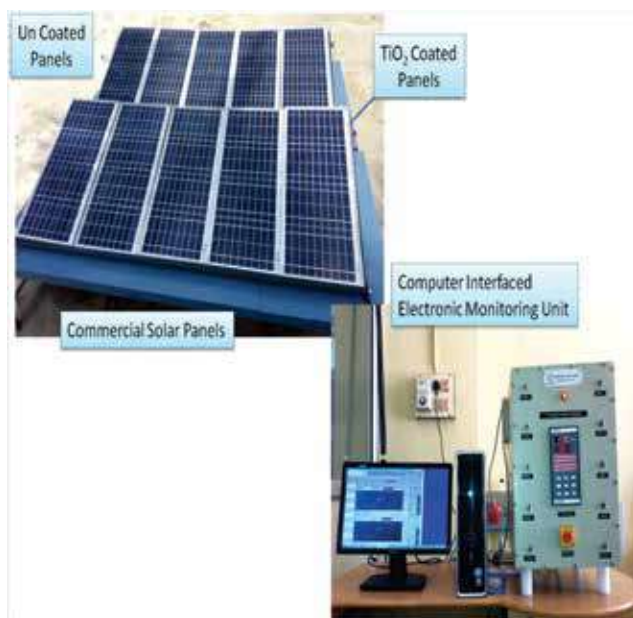
Fig. 2. Demonstration set up installed in NIIST
